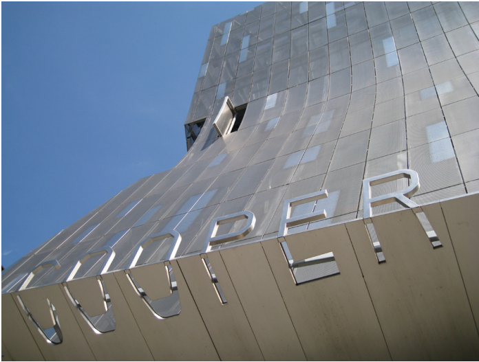
Figure 4. The façade of 41 Cooper Square, by Thom Mayne reveals hazy rectangles through the use of Zahner's perforation system.
