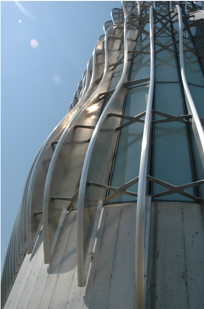
Figure 3. Zahner's headquarters, structural fins without metal panels. Also shown is the curved profile of the flange, forming a D shape. This shape allows panels to attach at any angle along the circumference.
