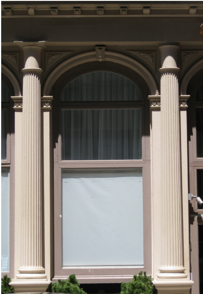
Figure 2. 85 Leonard Street detail. Note partially engaged columns.
